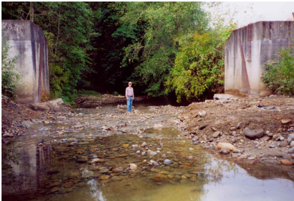
Landowner, Mike Danielle standing in creek after removal of concrete apron, stream restored to natural channel level
